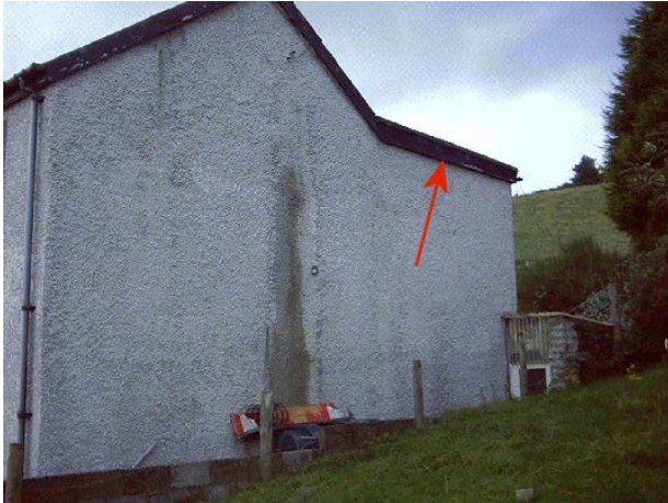
Figure 9. Roost at a barge board © Austin Hopkirk
