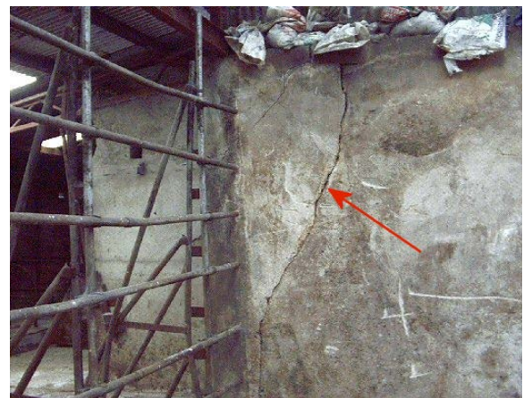
Figure 8. Wall roost in a crack © Austin Hopkirk
